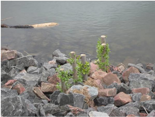
(7) continuous development of willow log branch cuttings; April 2012
