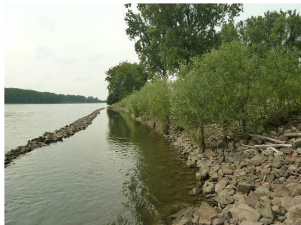
(12) willow log branch cuttings 2 ½ years after installation; May 2014
